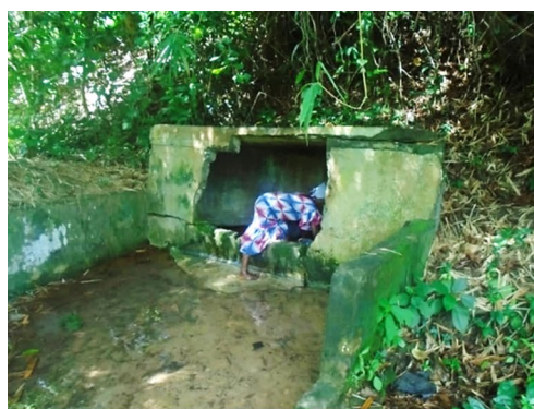
Fig. 6 Example of backwater improvement in Gbiéguhé and Gboguhé (Source: Field survey, 2022)
